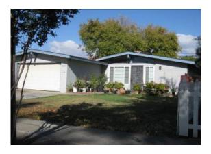
Figure 25 Flat or Minimally-Sloped Roof Source: Jose Villareal
