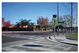
Figure 20 ADA Compliant Sidewalk
