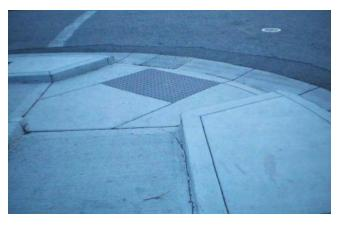
Figure 22 ADA Compliant Ramp
