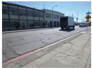
Figure 18 - Poor Pavement Conditions near Wattling St.
