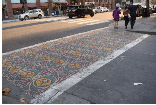
Figure 9: Pavement Design at the entrance of San Pedro Square Market
